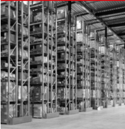
Pallet Racking - P90
