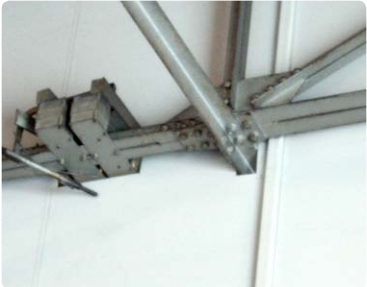
Sigma can be cut to accommodate an existing structure, providing an aesthetic finish.
